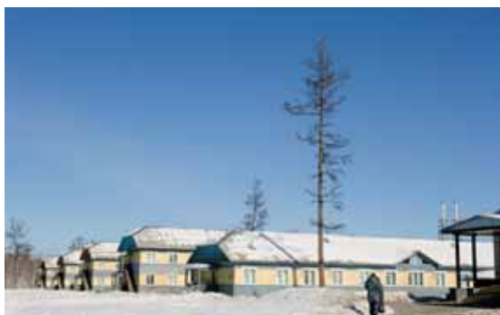
Accommodation camp at Pokrovskiy Rudnik
